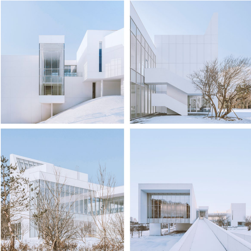
Exteriors of the building nearing completion, January 2024
