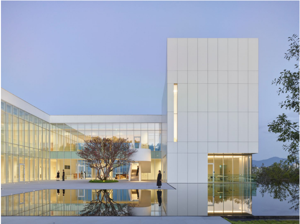
Central courtyard with reflecting pool, looking towards the “cube” and the transparent entrance and lobby pavilion Photography by Roland Halbe, October 2024
